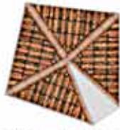
Church Tower roof
